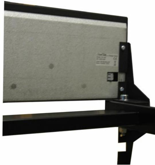
*Secure the CH-103 to the brackets using four 4mm screws. Run the power cables through the conduit down to the power supply*
